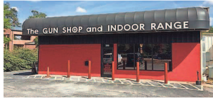
Bollards were installed at The Gun Shop in Simpsonville following a burglary in which a stolen minivan was intentionally crashed into the front.
